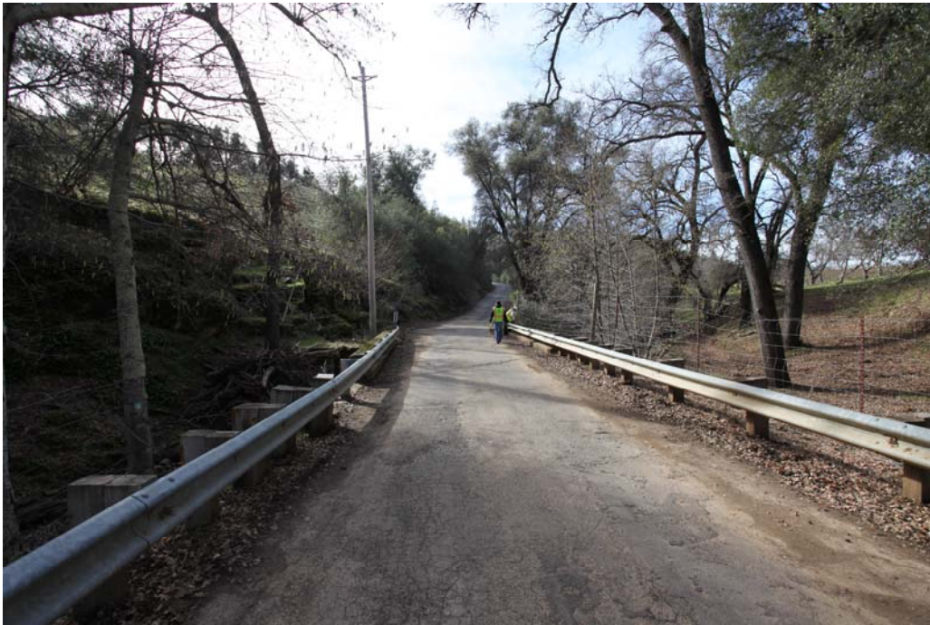
Looking South along Dogtown Road
